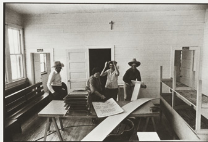
Community project of renovating a hall
